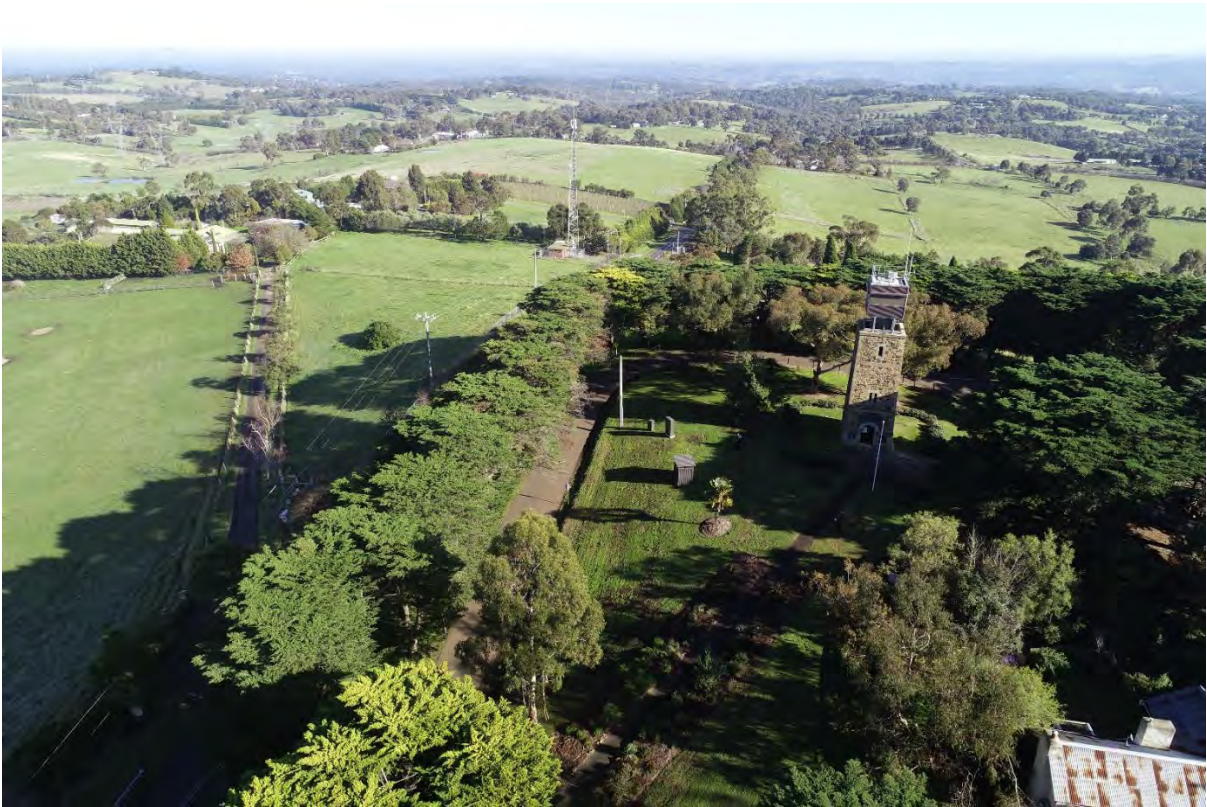
Heritage listed perimeter cypress trees are in a state of decline
