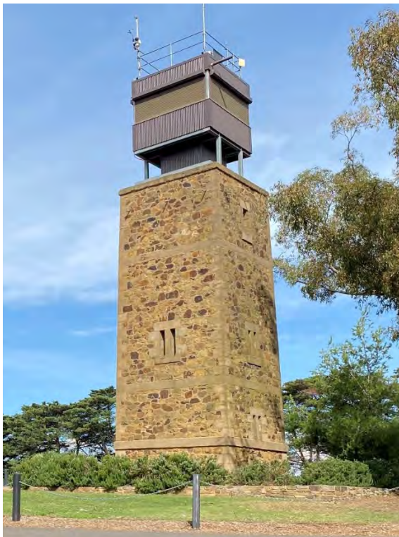
Fire-spotter's cabin on top of the tower
