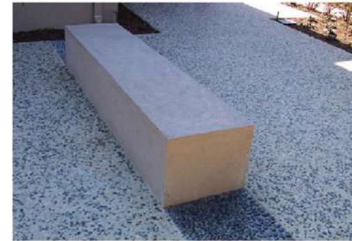
An example of in situ concrete walling
