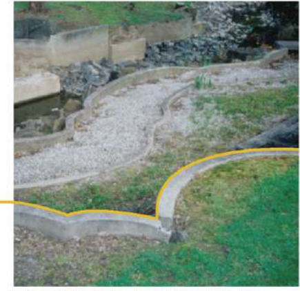
Existing retaining walls in the Old Hat Factory garden
