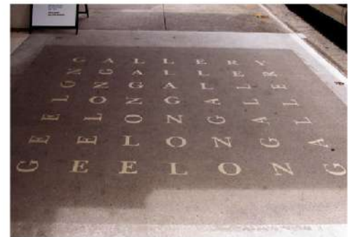
Utilising paving paint and stencils for pavement detailing
