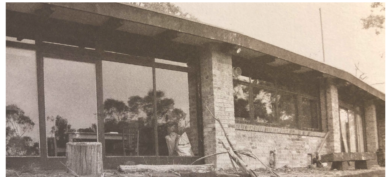
Previous page: Birrarung House. Image: John Gollings AM 2020 Opposite: Birrarung house and studio. Image: Eugene Howard 2019 River Bend House (formerly Cuming House) designed by renowned architect Alistair Knox. Image: Jane Woollard
