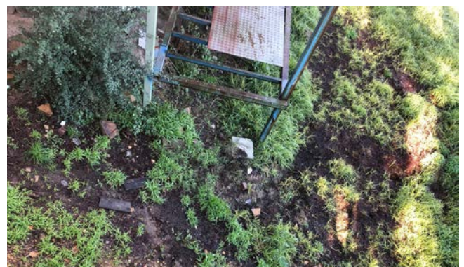
Figure 3: Wastewater overflow at a property in North Warrandyte
