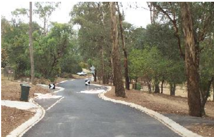
URBAN RESIDENTIAL ROAD CONSTRUCTION
