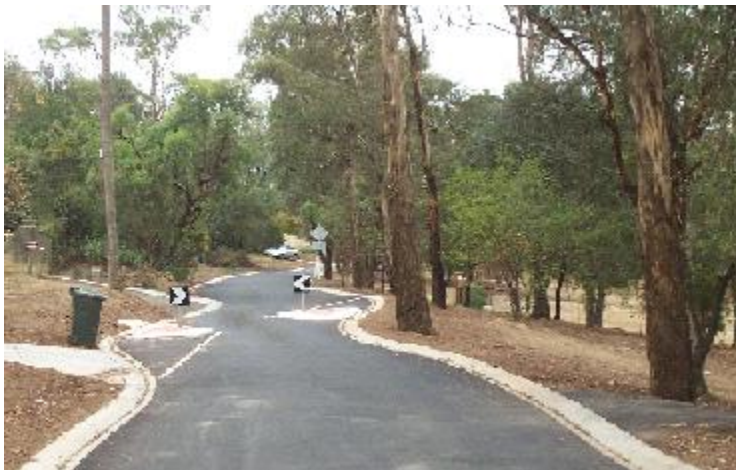
URBAN RESIDENTIAL ROAD CONSTRUCTION
