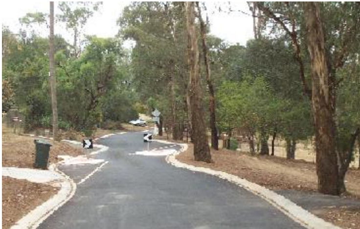
URBAN RESIDENTIAL ROAD CONSTRUCTION
