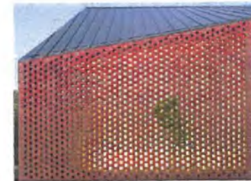
Precedent "Hit and Miss" brickwork Colour: Chapel Red Image: Nubrick Austral Bricks
